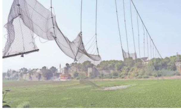
The bridge collapse in October 2022 killed 135. File
