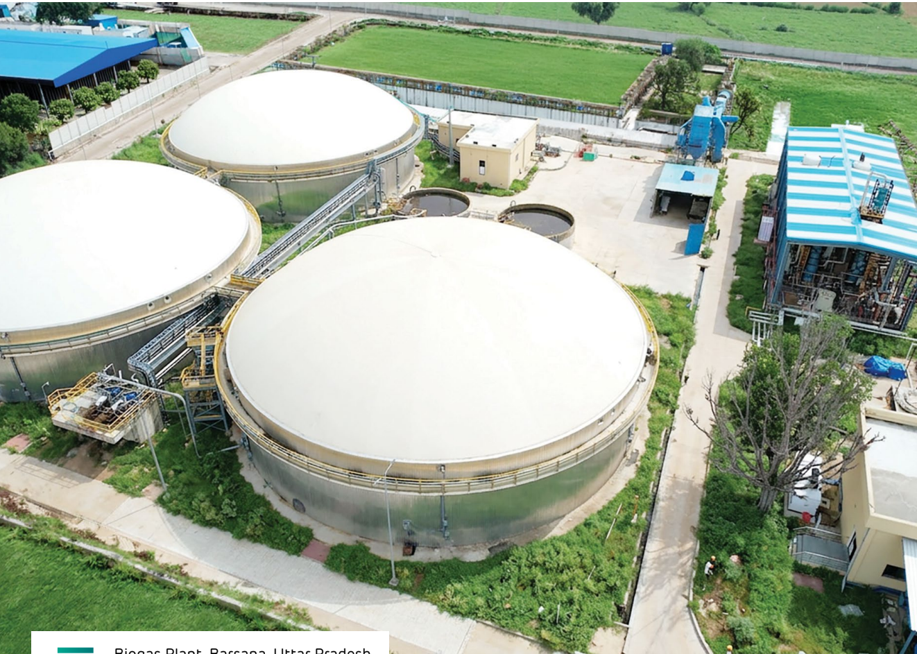
Biogas Plant, Barsana, Uttar Pradesh
