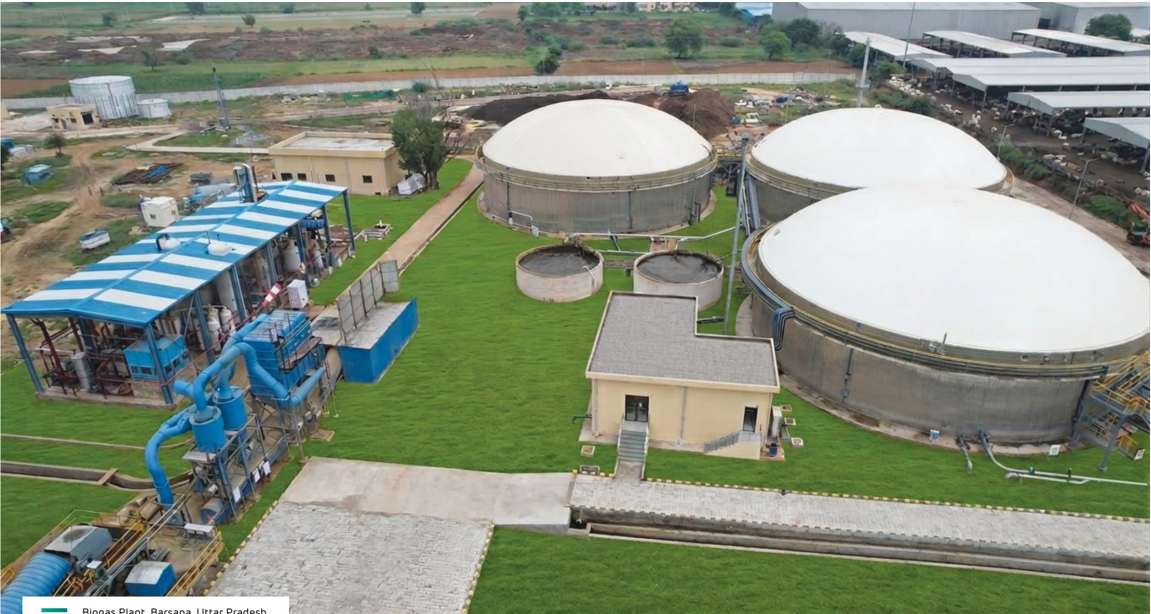
Biogas Plant, Barsana, Uttar Pradesh
